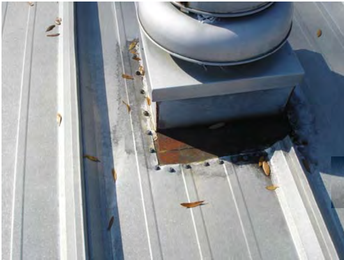
Existing Roof Penetrations
