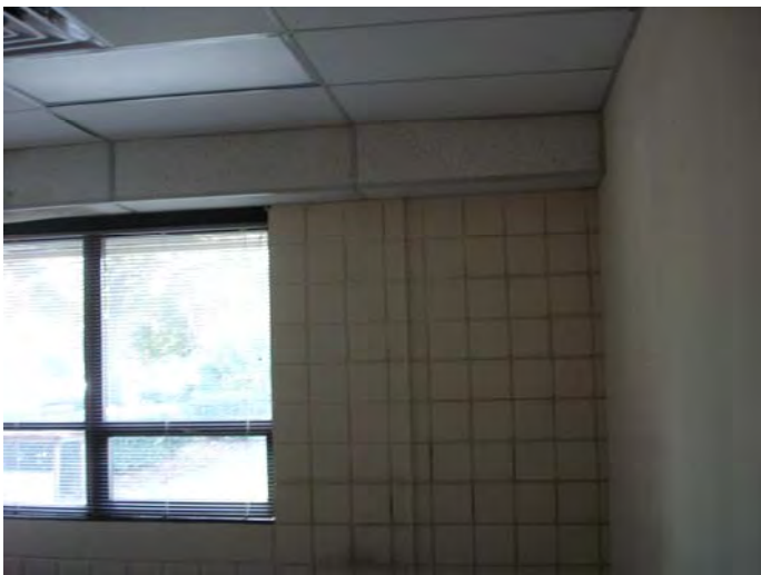
Block Wall and Typical Fenestration
