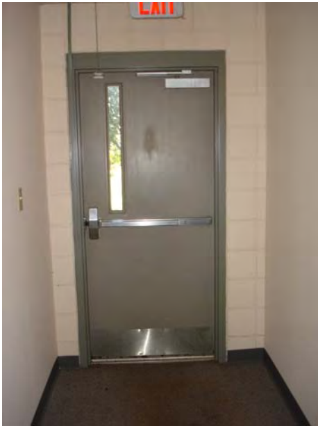
Existing Exit Door
