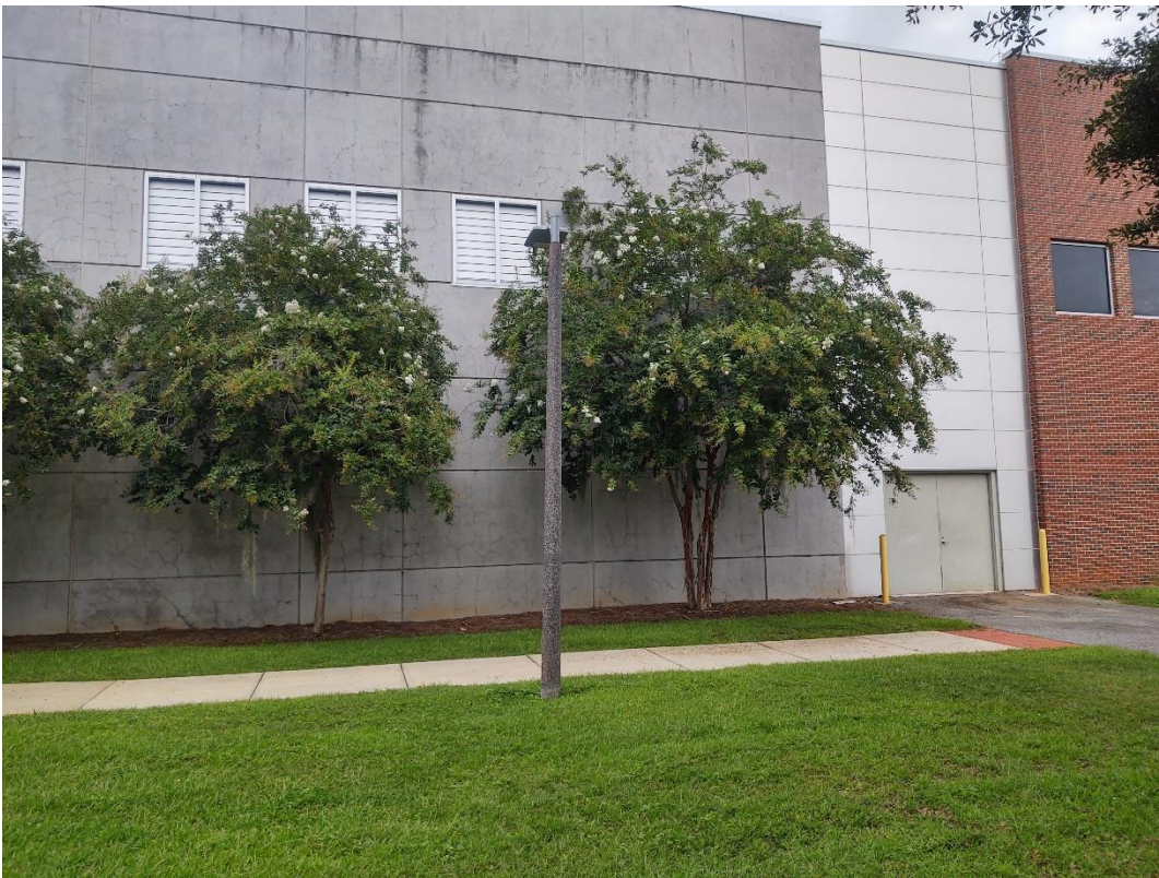
Existing East Exterior Elevation – AME Building
