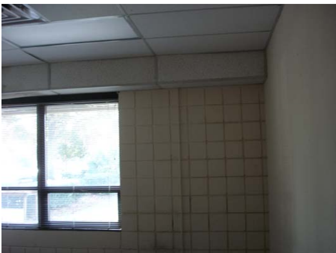
Block Wall and Typical Fenestration
