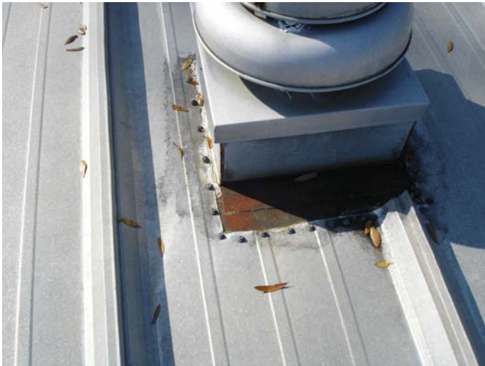
Existing Roof Penetrations
