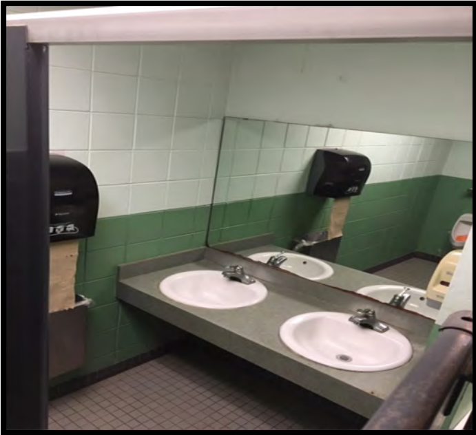
MENS RESTROOM BEFORE
