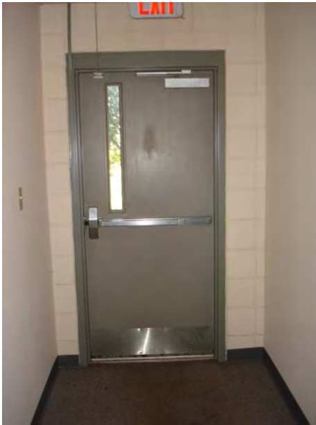
Existing Exit Door
